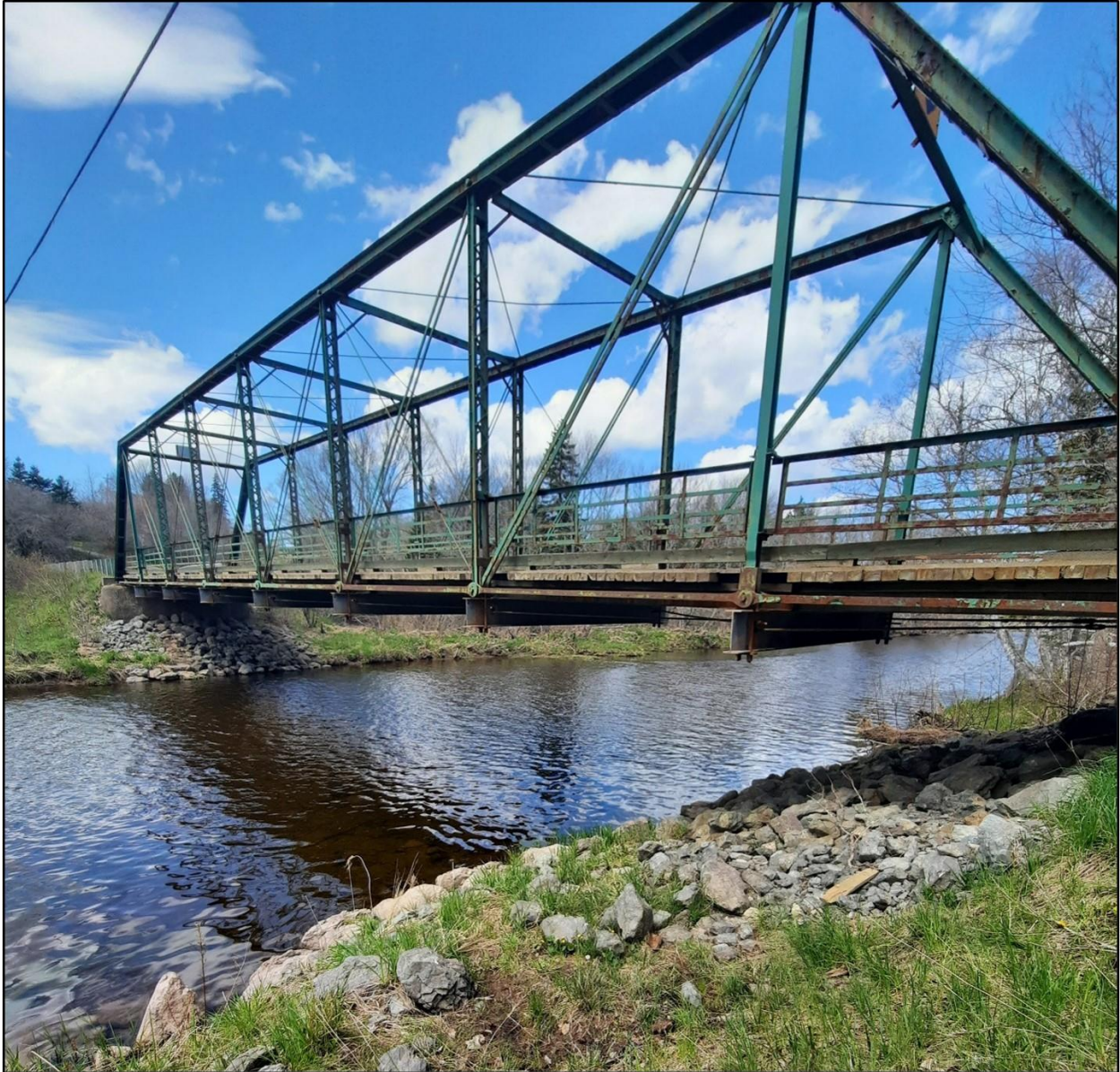
Figure 93: Blacksmith Valley Road crossing over the South River
