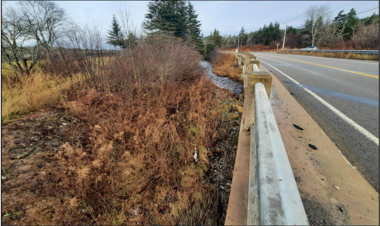
Figure 96: Upper South River Highway 316 road crossing (above)
