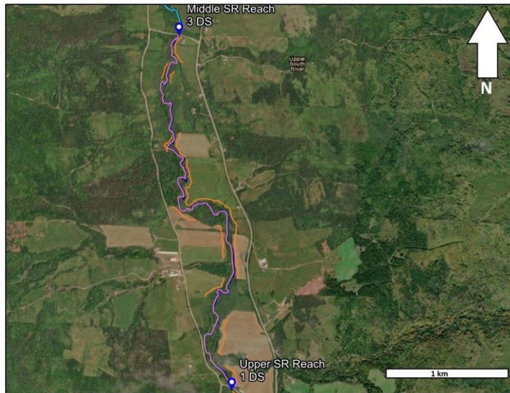
Figure 20: Aerial map of Reach #3. River highlighted in pink and bank lacking riparian zone highlighted in orange
