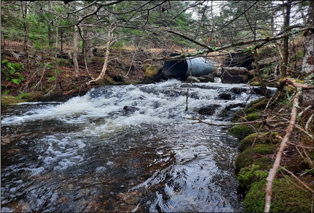
Figure 94: Argyle Road culvert downstream view
