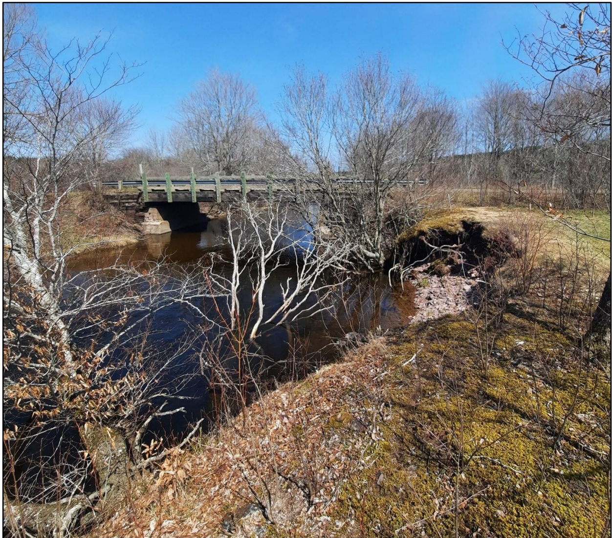
Figure 51: Looking downstream at the Cumming Mills Crossing Road bridge
