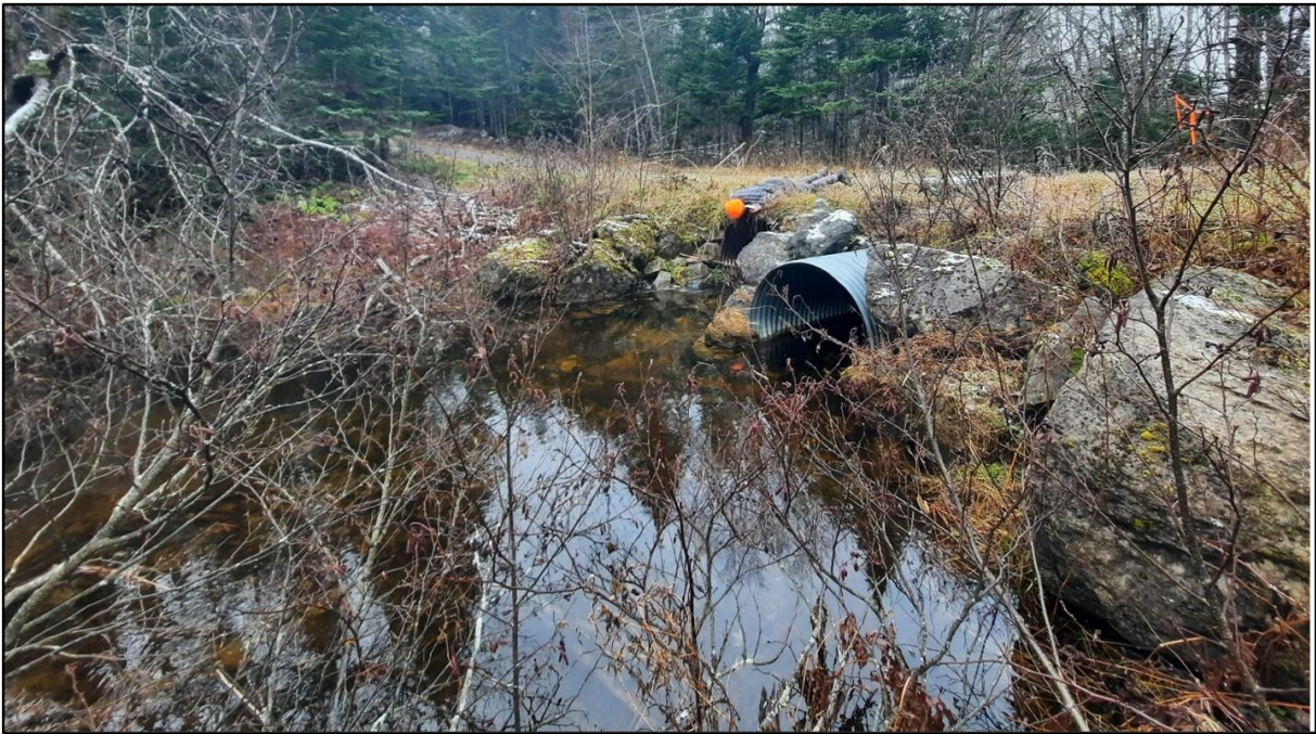
Figure 95: Argyle Road culvert upstream view
